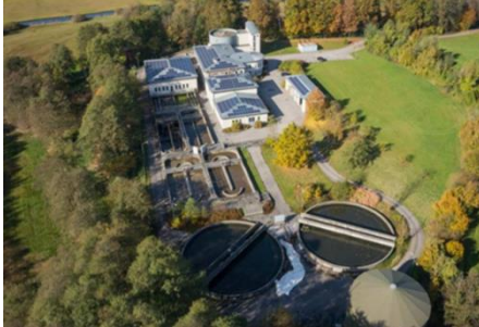
WWTP TRUMERSEE (A)
