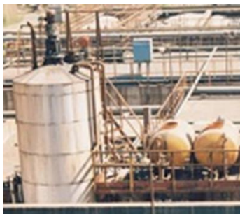
COKE PLANT ZENICA (BIH)
