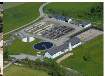
WWTP NEUMARKT (A)
